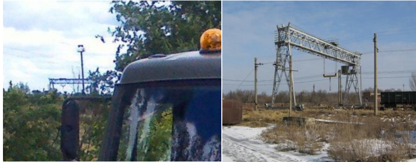
Left: gantry or portal crane visible on Dmitry's photograph in the distance behind a floodlight tower. Right: gantry crane type KK 30-32, similar to the type of crane in Dmitry's photograph.
