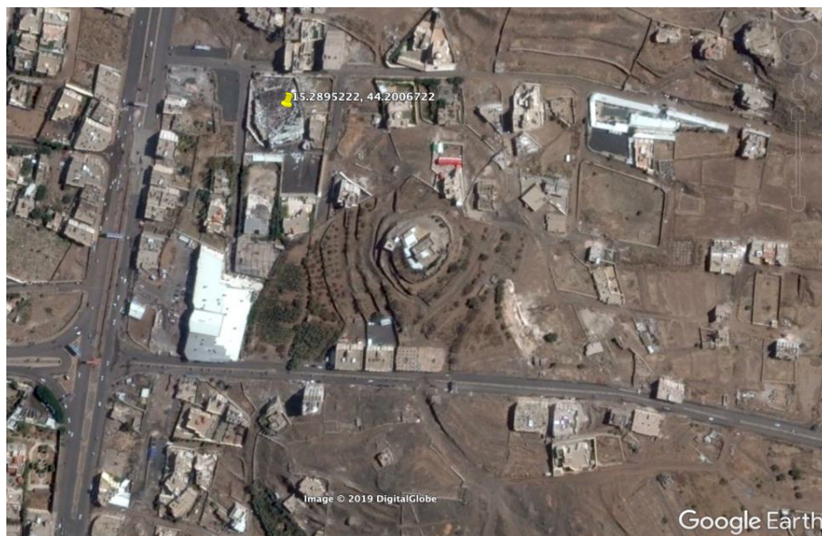
A satellite image showing a destroyed building at the site of the airstrike on 04/02/2019 (Courtesy of Google/Digital Globe).
